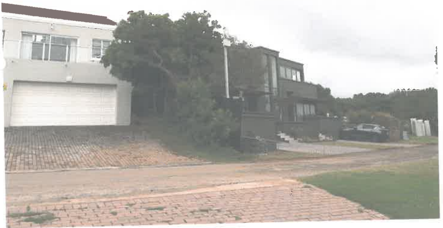
View of Existing Structure 2
