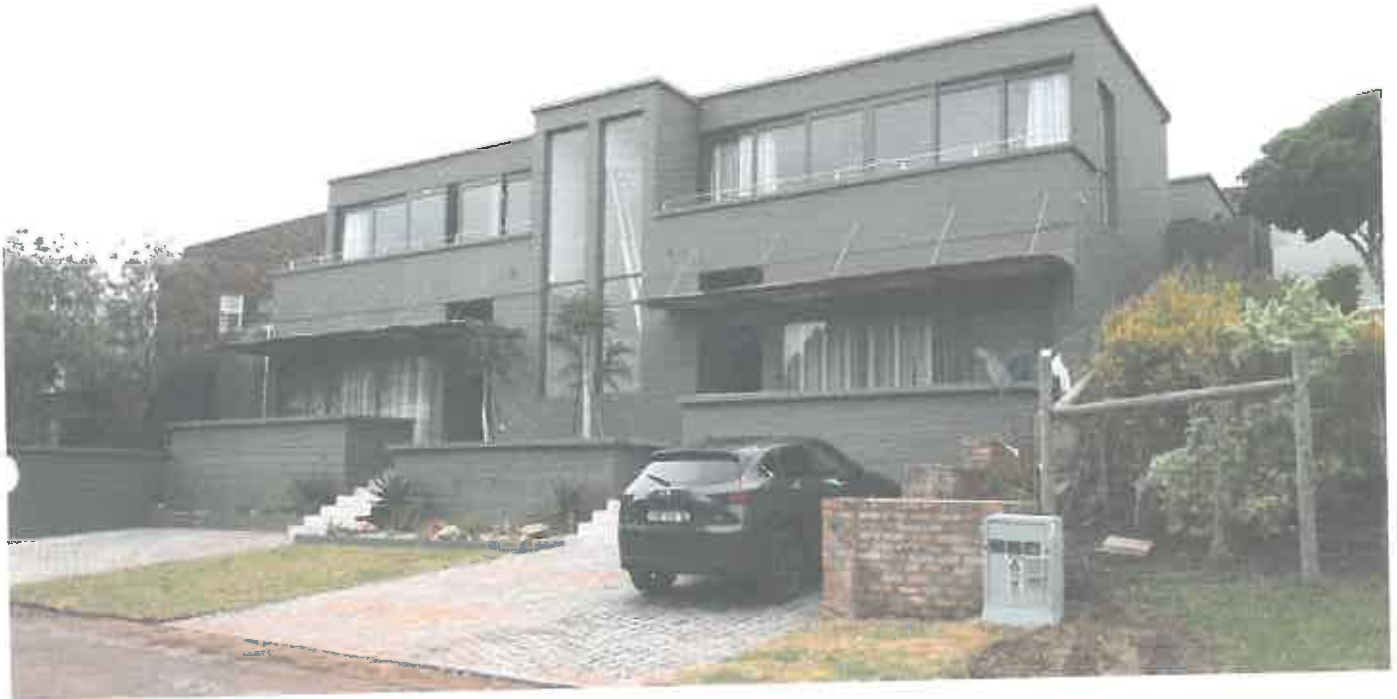
View of existing structure 1
