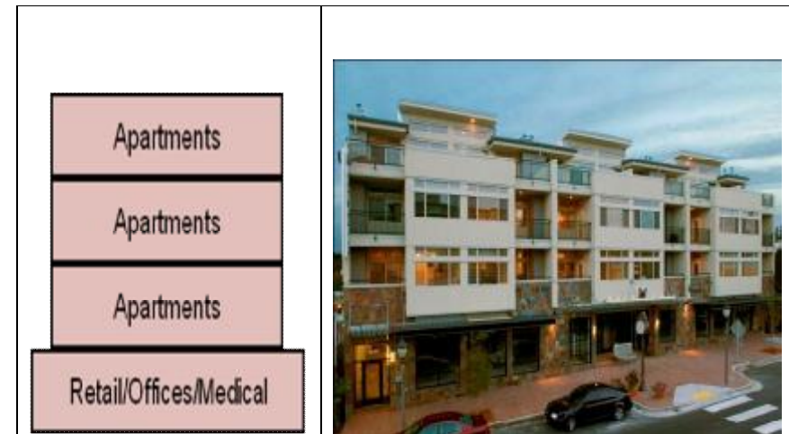
Figure 24: Example of Mixed use development
